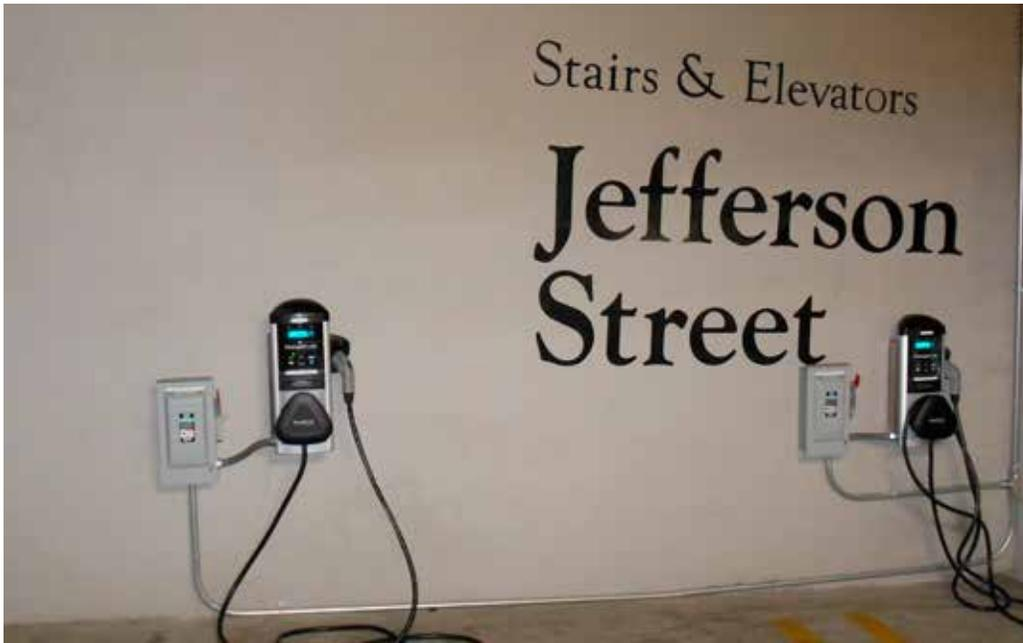
With the energy reduction from the lighting enhancements, ABM also was able to increase the facility's power capacity and installed several ChargePoint® EV charging stations, without the need to upgrade the facility's existing electrical system. This was an added bonus for the city.
