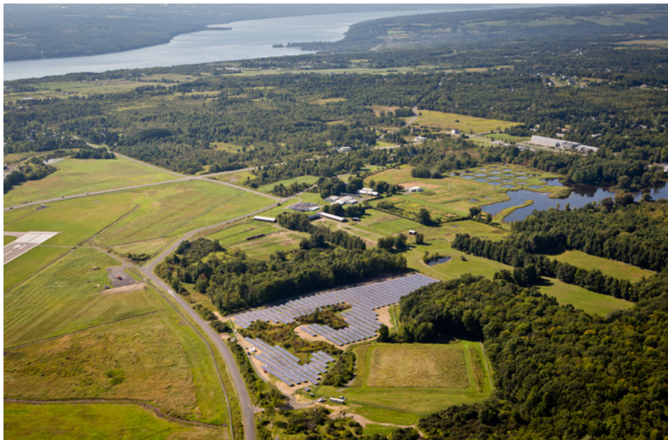
ABM EPC team installs 2MW solar array for Cornell University
