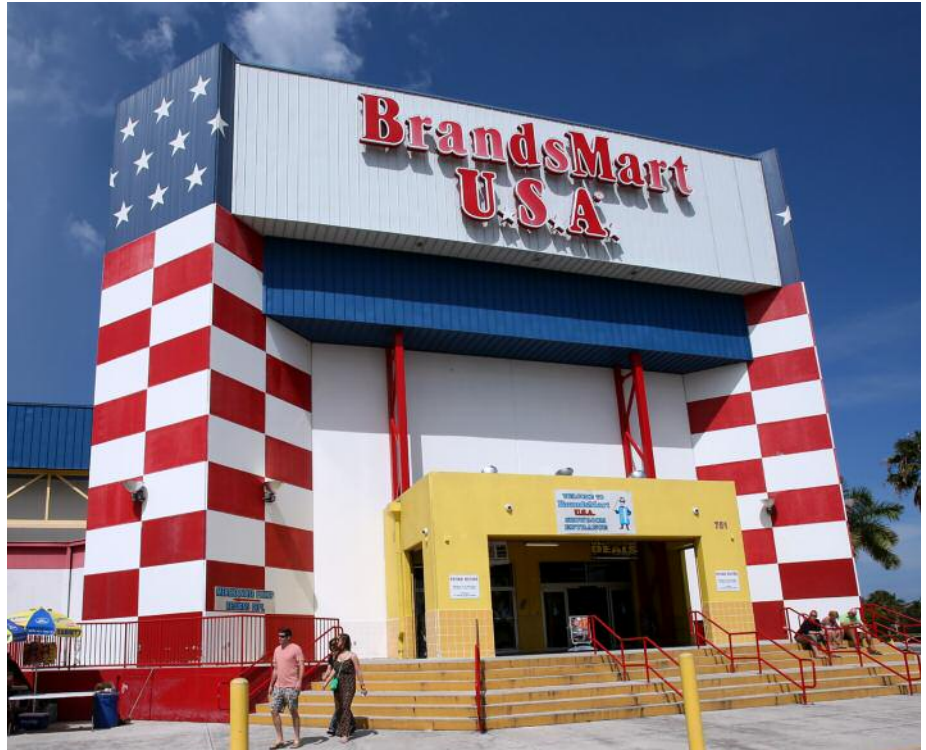
BrandsMart received $2.225 million from a private investor for an energy efficiency upgrade project. Facility management service provider, ABM, has managed the project for the retailer.
