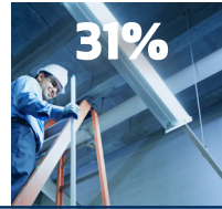
LED LIGHTING RETROFITS
